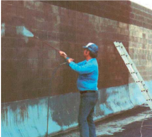
Surface Shield being applied to a concrete block sound barrier
